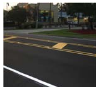
Brownswitch Road Improvements, St. Tammany Parish, LA
